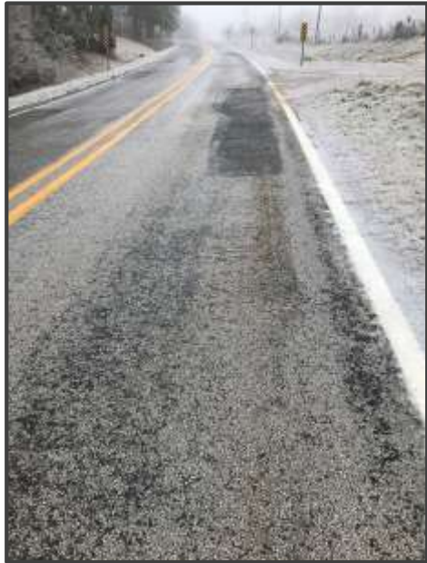
Newton County Highway 327 South of Jasper
